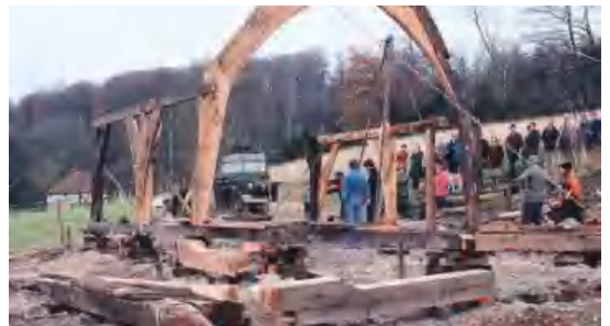
This photo from the 1970s shows the re-erection of the massive central 'cruck' frame timbers Photograph courtesy of Weald & Downland Museum Archive
